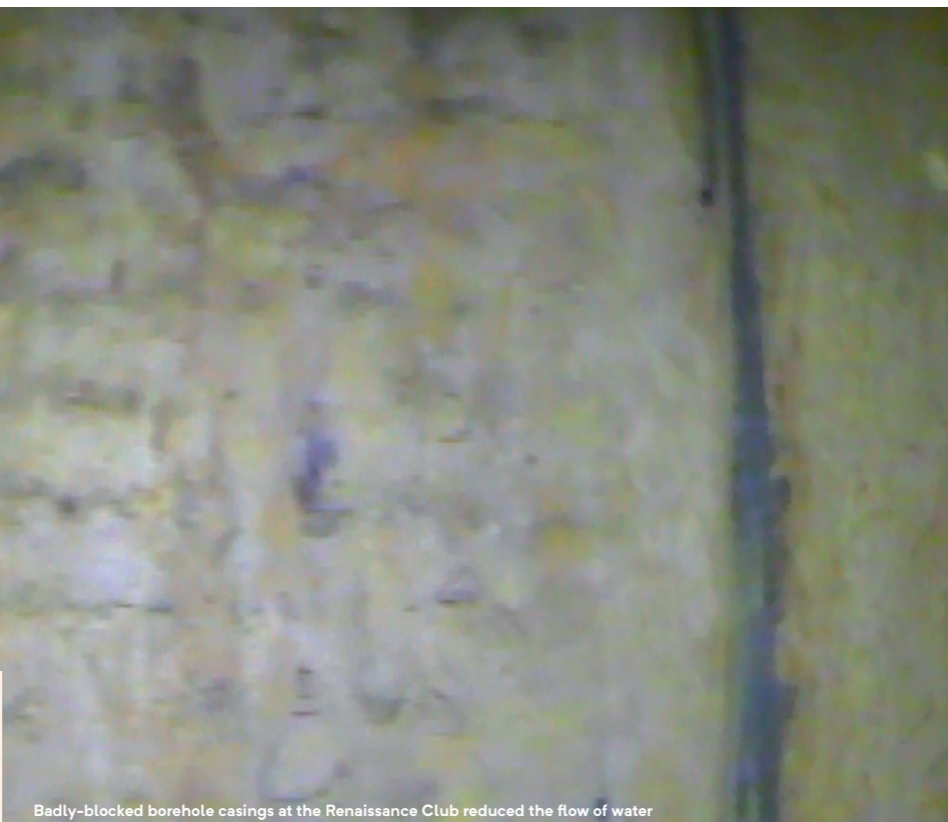
Badly-blocked borehole casings at the Renaissance Club reduced the flow of water
